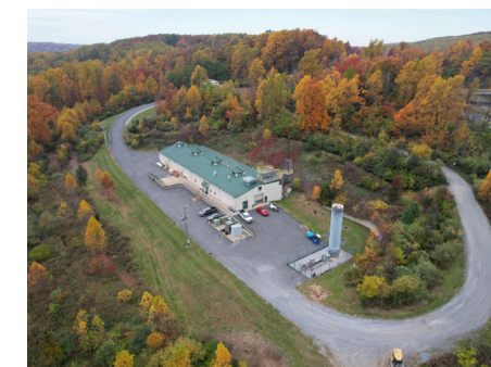
Morgan Town 20MW Pennsylvania, USA
