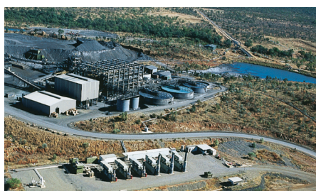
McArthur River Mine Power Station 77MW, Northern Territory, AU
