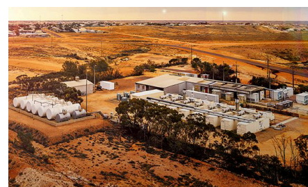
Coober Pedy Hybrid Renewable Power Station 9MW, South Australia
