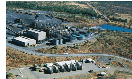
McArthur River Mine Power Station 77MW, Northern Territory
