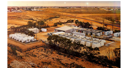
Coober Pedy Hybrid Renewable Power Station 9MW, South Australia
