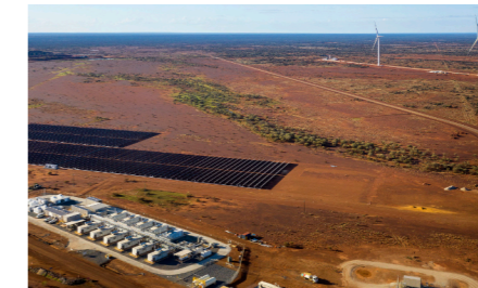
Agnew Hybrid Renewable Microgrid 60MW, WA
