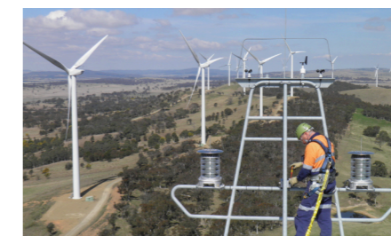
Cullerin Range Wind Farm 30MW, New South Wales
