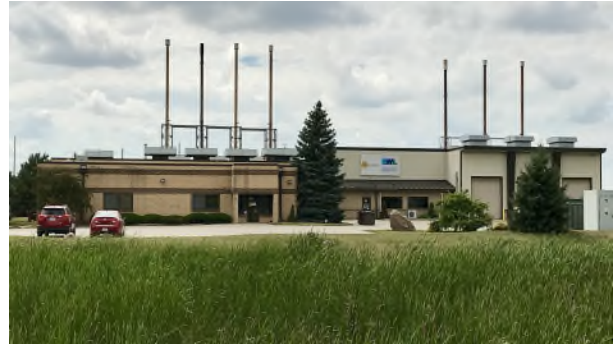
EDL's Wood Road RNG plant in Michigan, USA
