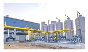
In a natural progression, EDL is developing RNG projects at several of our LFG power stations in the USA. Our Indy High BTU RNG Plant (pictured above) was commissioned in 2020. It is the largest in Indiana, USA with capacity to convert LFG to approximately 8 million gallons of pipeline-quality RNG each year.
