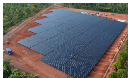
Weipa Solar Farm
