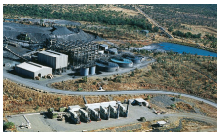
McArthur River Mine Power Station
