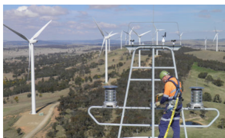
Cullerin Range Wind Farm
