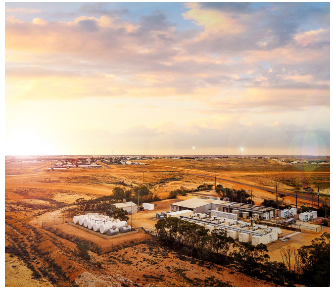
Coober Pedy Power Station
