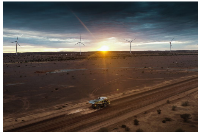
The Agnew Hybrid Renewable Power Station comprises wind, solar, gas and diesel generation and battery storage.
