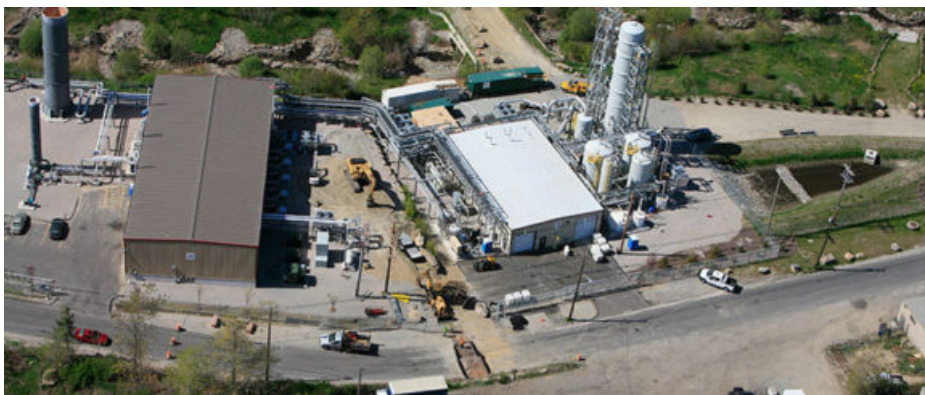
Johnston LFG Plant
