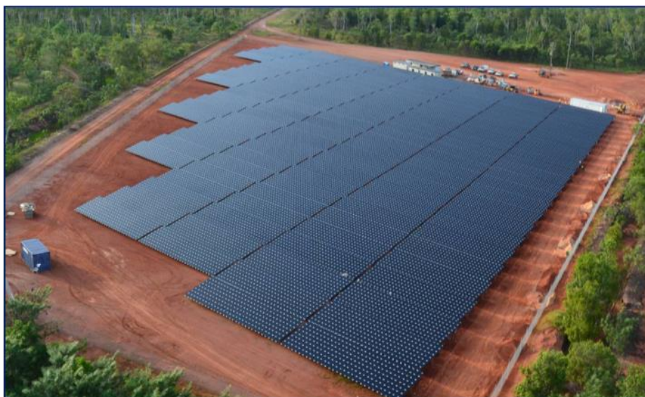
Weipa Solar Farm
