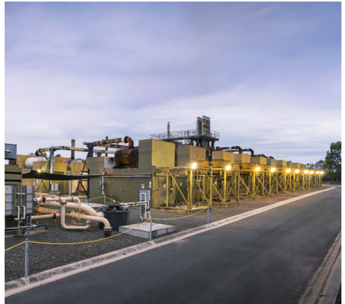
Lucas Heights II Power Station
