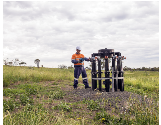
Lucas Heights landfill gas collection station
