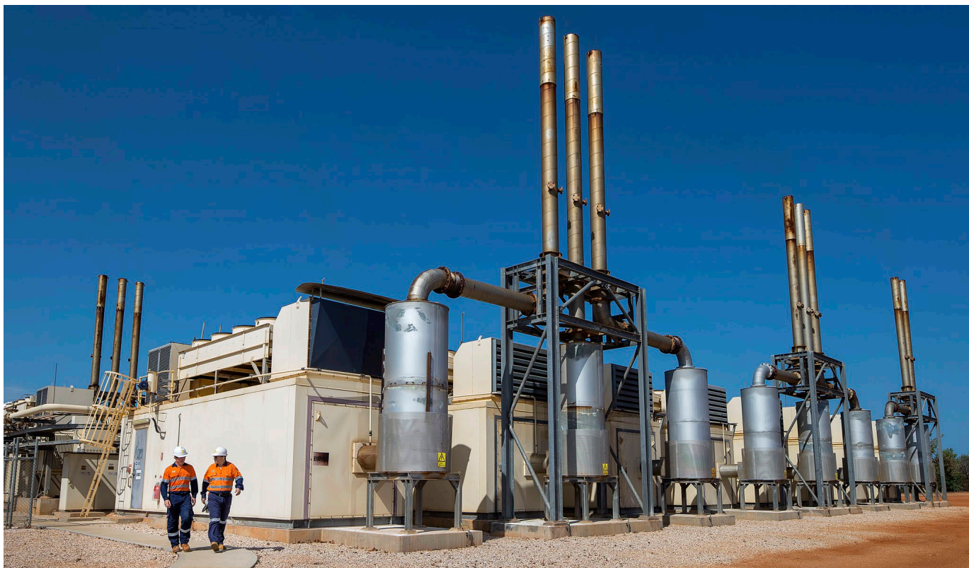
CAT3520C gas engines at Broome Power Station
