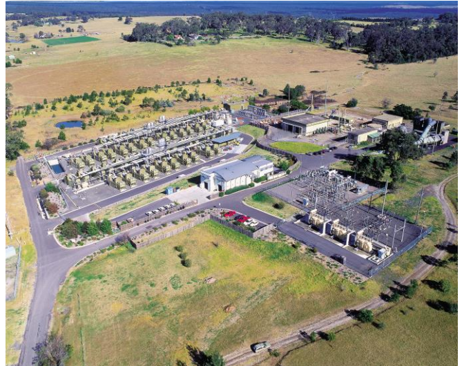
Appin Power Station
