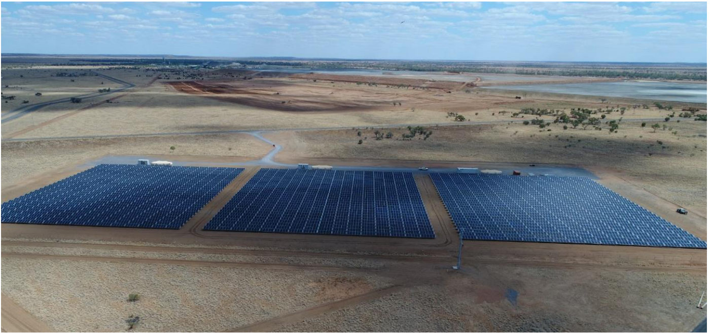
Solar PV facility at Cannington mine
